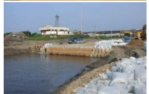
TEMPORARY JETTY CONSTRUCTION AT NAN-KAN RIVER MOUTH FOR KKPC POWER PLANT
